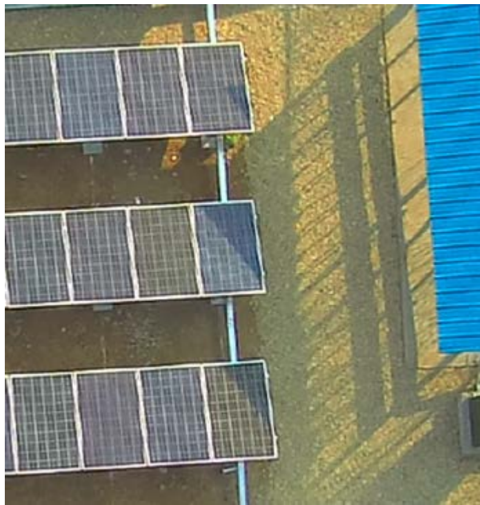
逆变器遮阳棚引起的热斑
